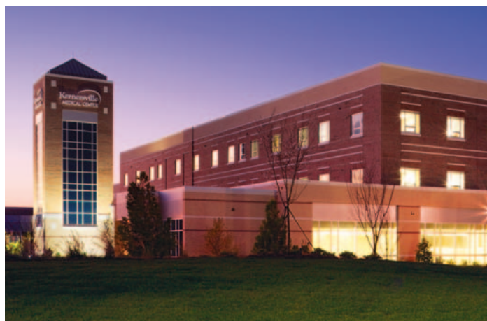
Kernersville Medical Center underwent the final phases of construction in 2010, and opened its doors to the community in March 2011.
